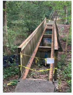
The cross beams on the bridge have been removed and plans are being made for a church work day to replace the foot boards.
